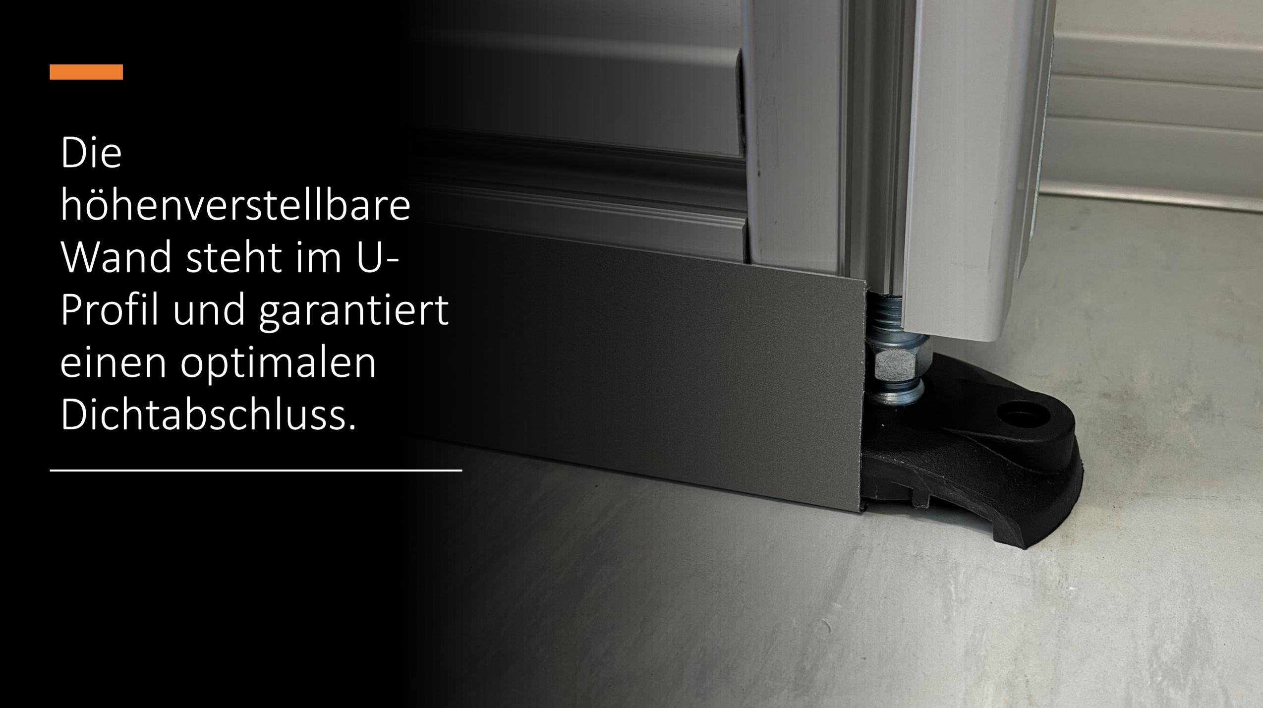
A close-up photograph showing the bottom edge of a grey wall profile. The profile is mounted on a black plastic base. A silver-colored metal screw is visible, which is used to adjust the height of the wall. The wall profile is shown in a U-shaped cross-section, and the text explains that this design ensures a tight seal.
